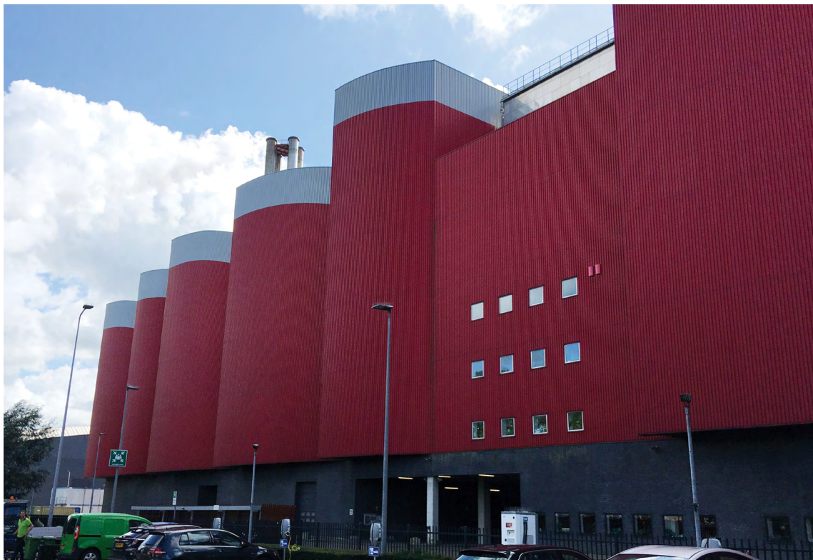
HVC, Waste to Energy Alkmaar, The Netherlands
