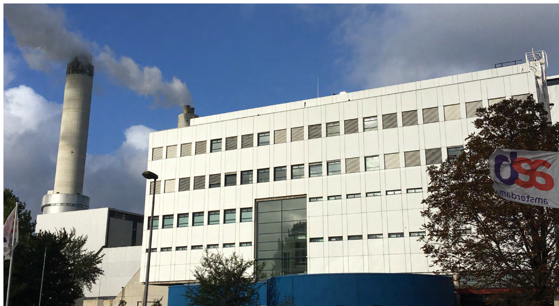
AEB Amsterdam Waste to Energy, The Netherlands
