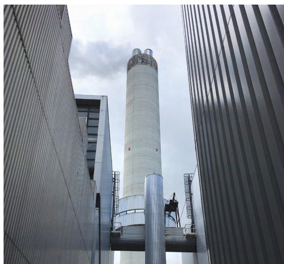
AEB Amsterdam Waste to Energy, The Netherlands
